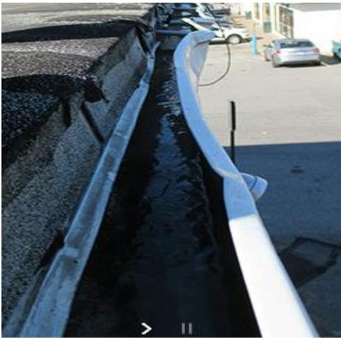
THIS RESIDENTIAL GRADE GUTTER ON A COMMERCIAL BUILDING HAS BEEN BENT AND DAMAGED.
